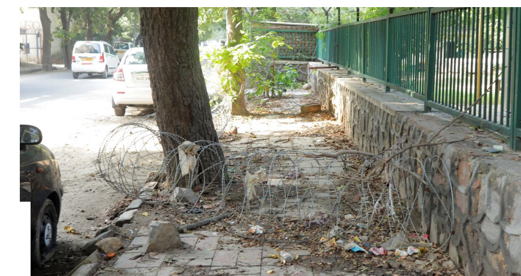
Obstructions on footpath: Ashoka Park road
