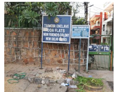
improperly placed signs
