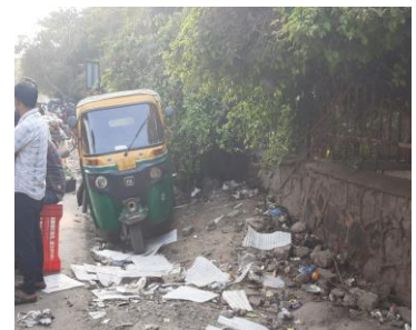
Broken and poorly maintained pathways
